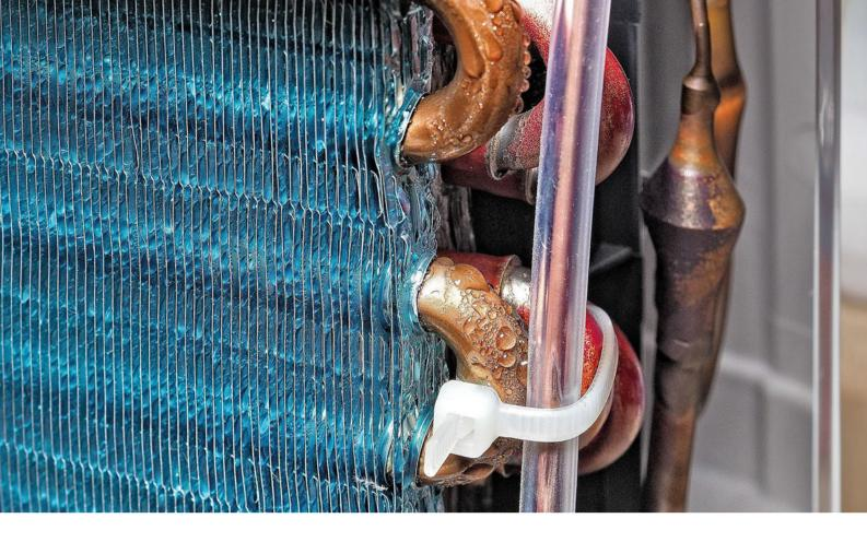
Refrigeration drying live: the room air that is taken in is cooled to below its dew point at the dehumidifier's cold evaporator and water condenses on the fins and refrigerant line.
