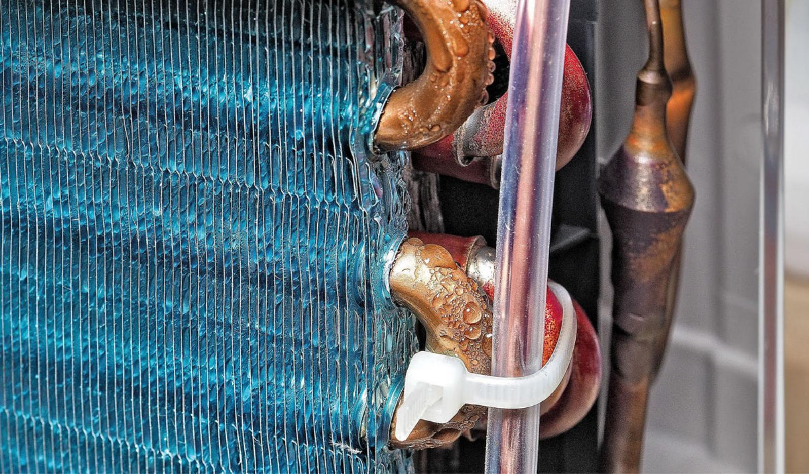
Refrigeration drying live: the room air that is taken in is cooled to below its dew point at the dehumidifier's cold evaporator and water condenses on the fins and refrigerant line.
